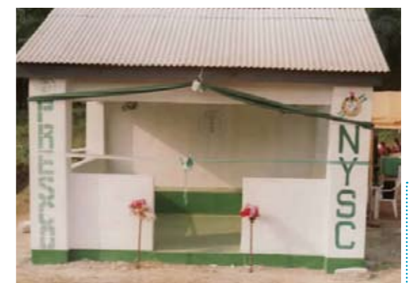
The bus stop shelter
